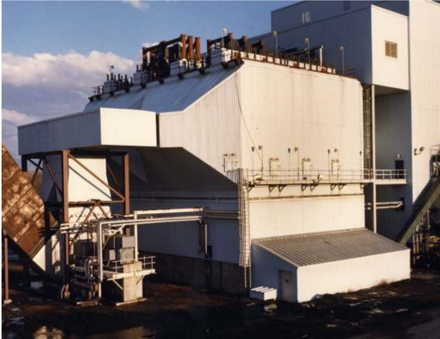
Burlington Electric, J.C. McNeil Station, Burlington VT
